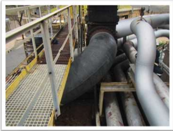
Figure2: The completed laminate repair solution.
