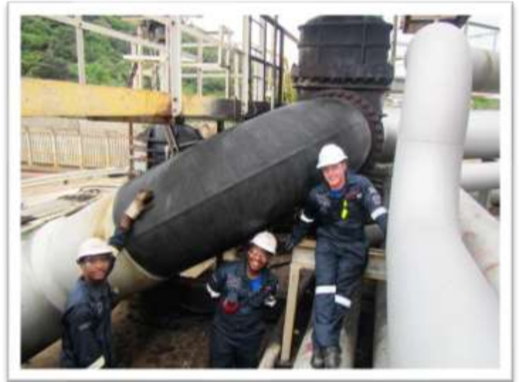
Figure 3: Contractor: Beruseal Pty Ltd
