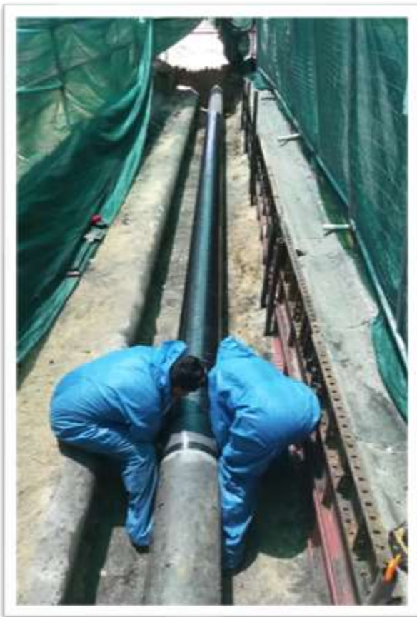
Figure 2: Application of the carbon fibre composite laminate repair system.
