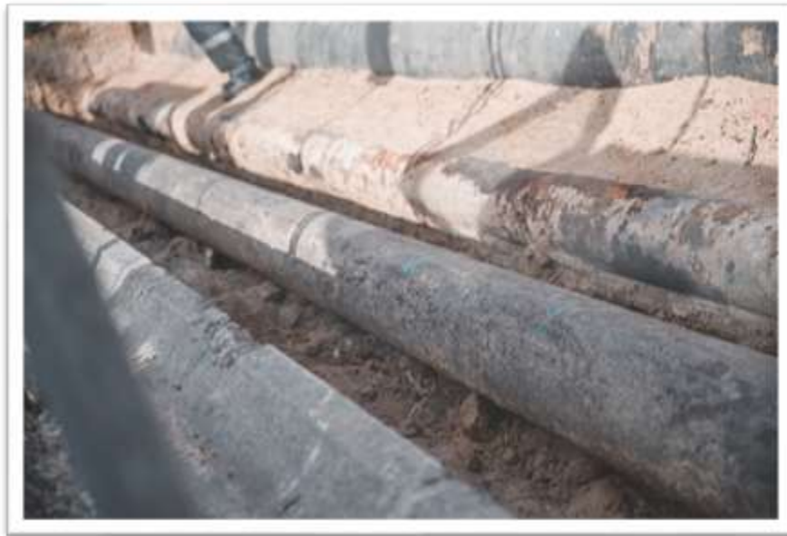
Figure 1 Excavated white oil straight pipe section.
