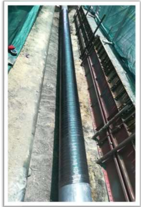
Figure 3: Completed carbon fibre composite laminate repair solution.
