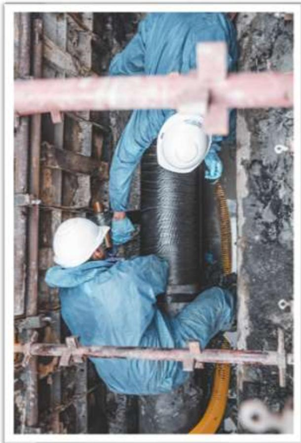
Figure 3: Peel-ply application as surface preparation for future adjacent repair wraps.
