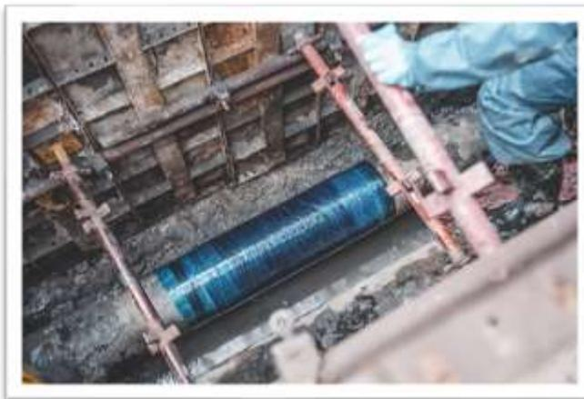
Figure 4: Application of compression film to uniformly distribute the resin by pressure.
