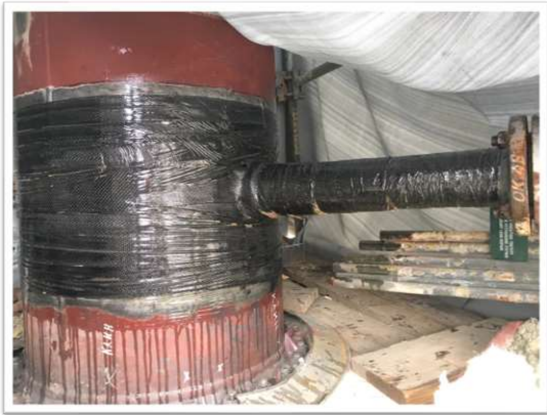
Figure 3: The final repair completed
