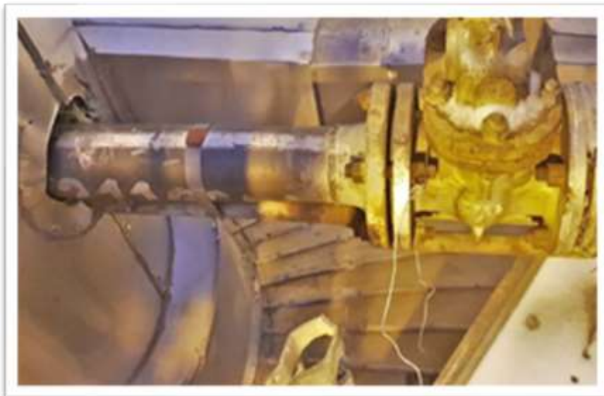
Figure1: Illustrating 2" take off with insulation still attached.
