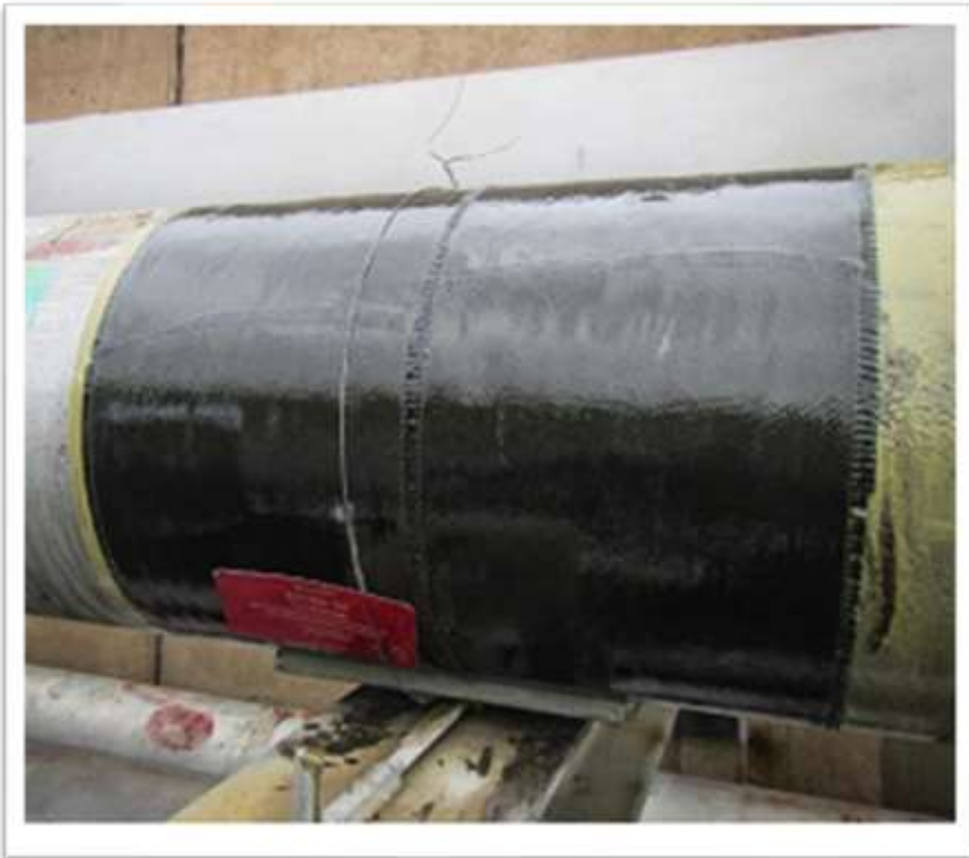
Figure 2: Shows the completed composite repair
