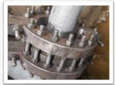
Figure 5: Bolted flange clamp prior wrap
