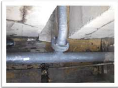
Figure 3: SSPC SP3 surface preparation of the elbow tee with flange.
