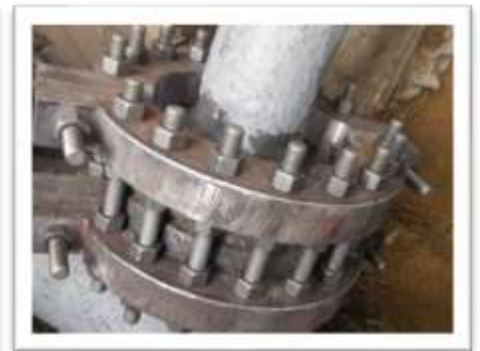
Figure 5: Bolted flange clamp prior wrap
