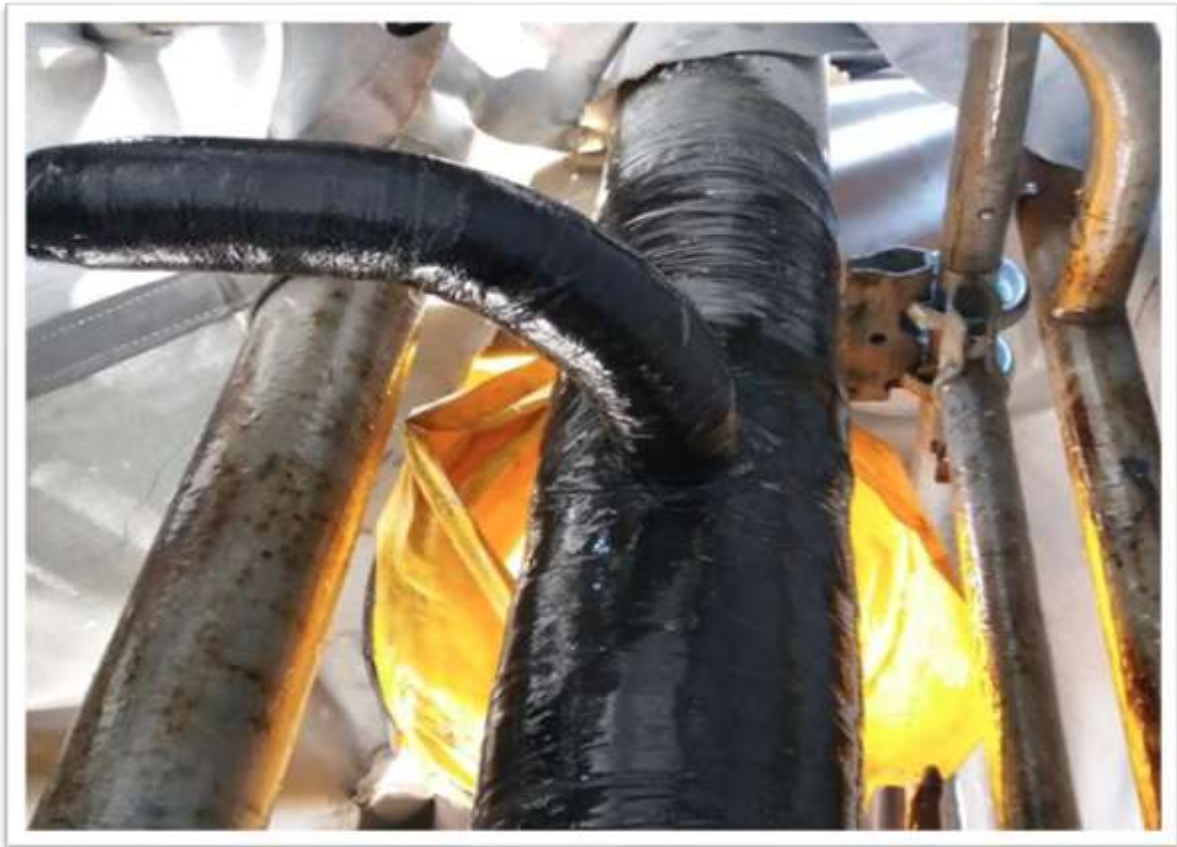
Figure 4: Curing in progress
