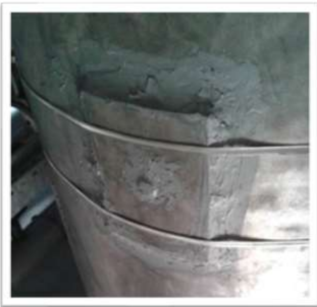
Figure 4: Patch secured with Revofill
