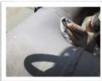
Figure 3: Surface Prepared for patch
