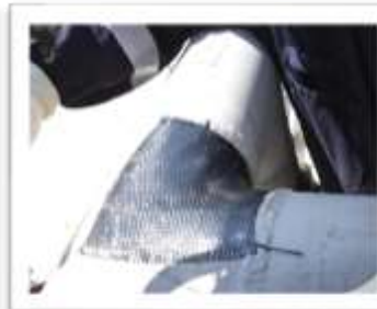
Figure 4: 2 x layers Revowrap 110 applied to create patch
