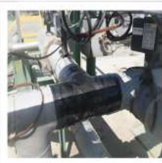
Figure 9: Completed Wrap
