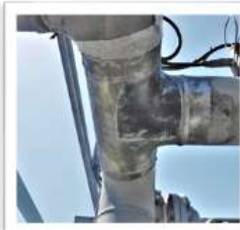
Figure 8: Patch applied
