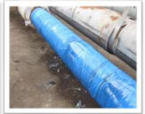
Figure 5: Revostretch applied to consolidate wrap
