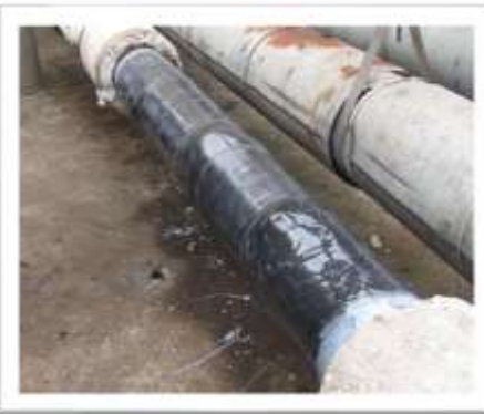
Figure 6: The Revostretch was removed after cure was reached
