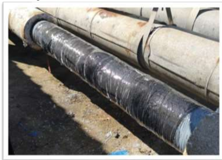
Figure 6: The Revostretch was removed after cure was reached
