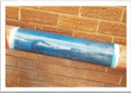
Figure 3: Pipe is Primed for wrap
