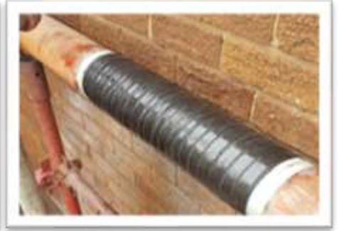
Figure 4: Completed wrap
