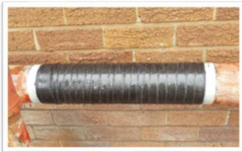
Figure 5: Completed wrap
