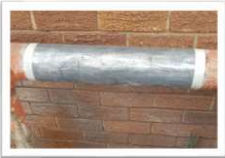
Figure 2: Surface prepared to SA2.5
