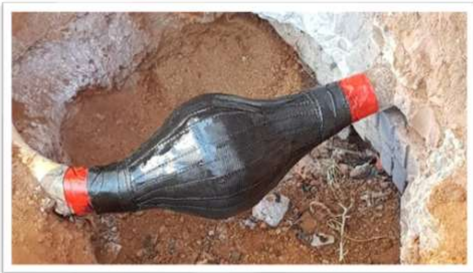
Figure 6: Axial strips of Revowrap was applied to cover the entire flange
