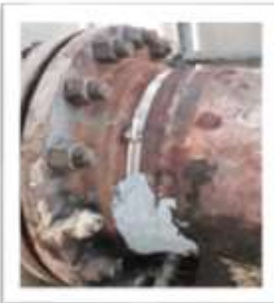
Figure 6: Hole repair with Revofill
