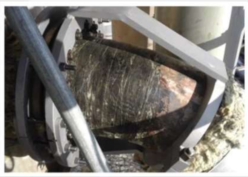
Figure 8: Wrap with Strongback installed
