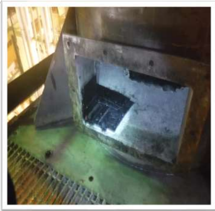
Figure2: Installed composite Internal wrap repair on manhole via patch repair.
