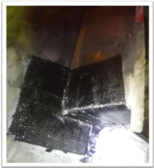
Figure 3: Installed composite External wrap repair on manhole via patch repair
