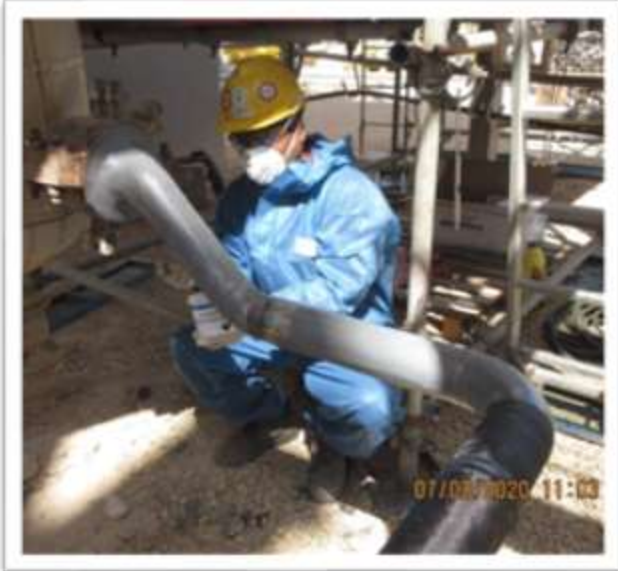
Fig 1: Primer being applied
