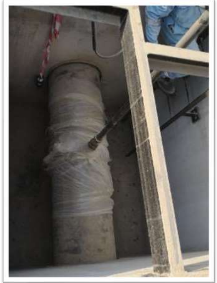
Fig 2: Overview of Repair area
