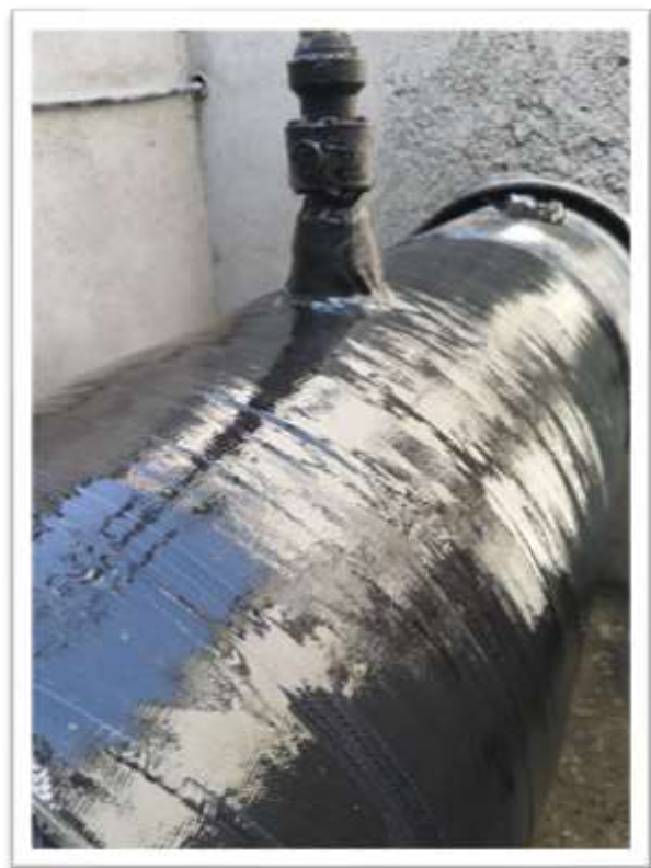
Fig 5: Completed wrap close up
