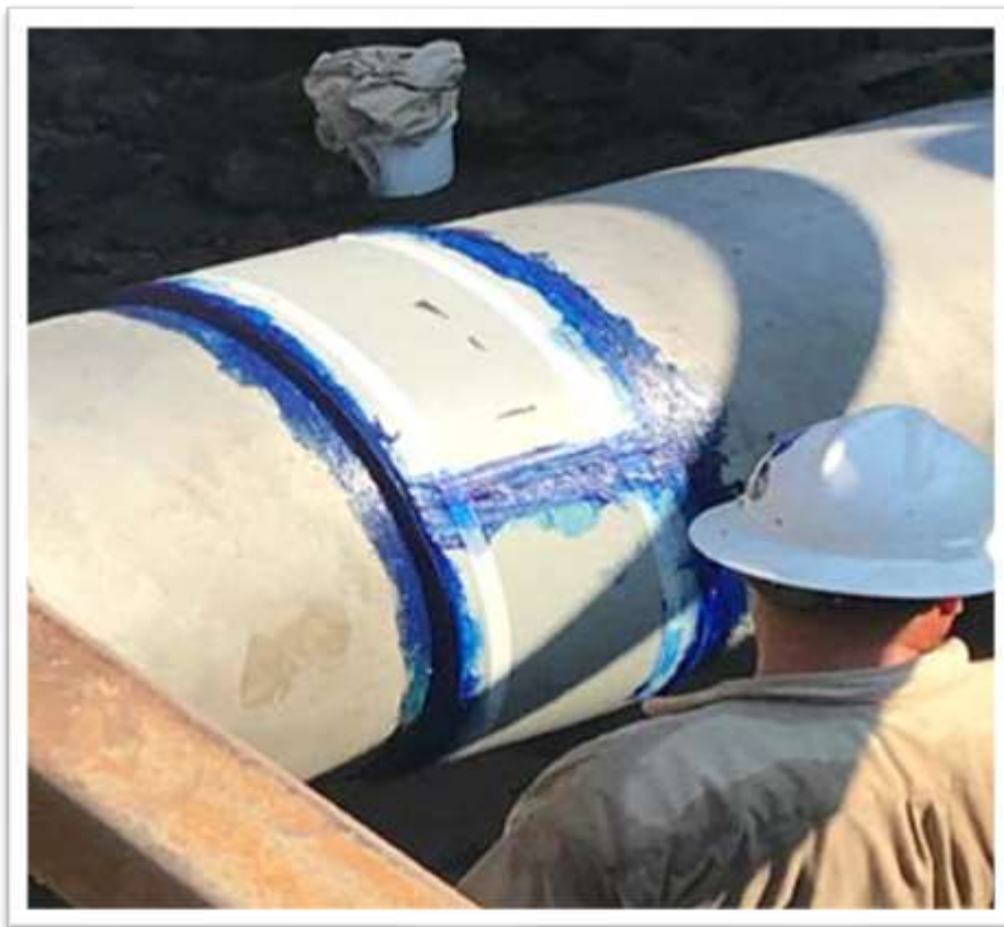
Fig 3: Completed Repair WITH "WELDWRAP"
